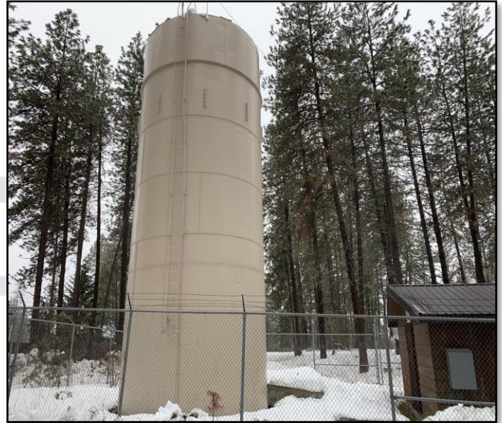
Fresh Paint on the 50,000 Gallon Reservoir
