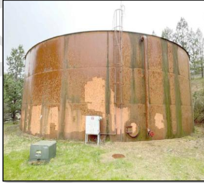
Ponderosa Tank Before and After Recoating
