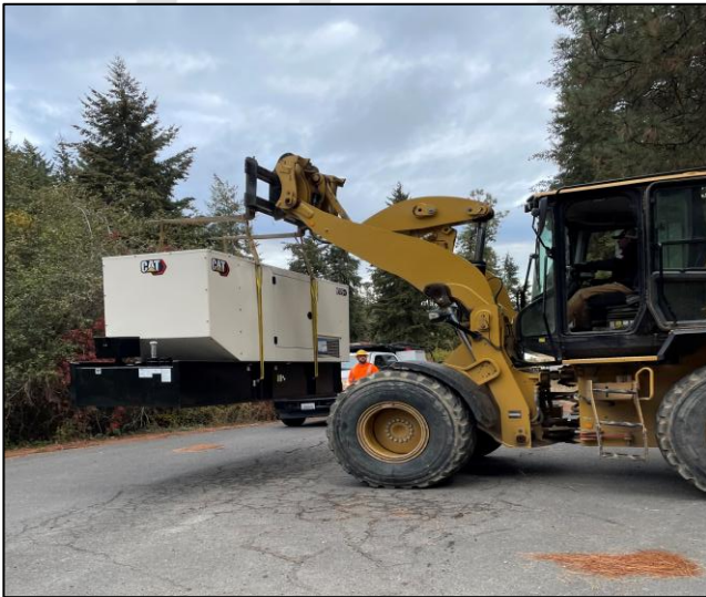
Crews Delivering and Installing a Fixed Place Generator at Horizon Hills Booster Station to Serve the Painted Hills Area
