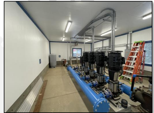
4 New 30 HP Motors and 1 New 10 HP Motor Inside the Florida Booster Station
