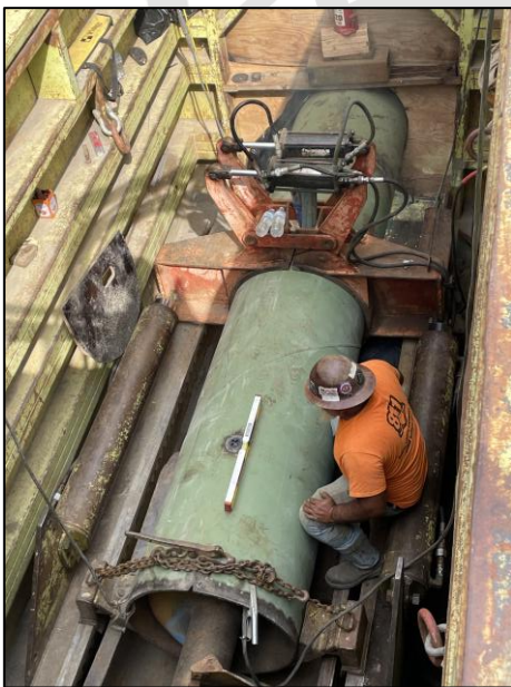
Contractor Pushing 30 Inch Steel Casing Under Hastings Road
