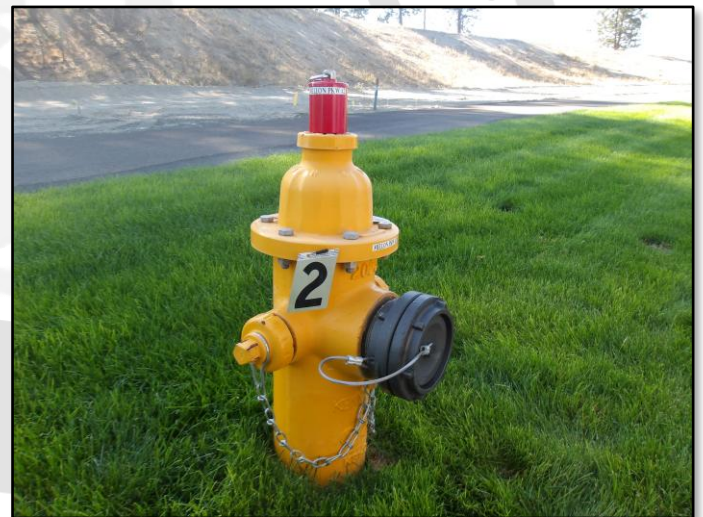
Locked Hydrant to Prevent Misuse
